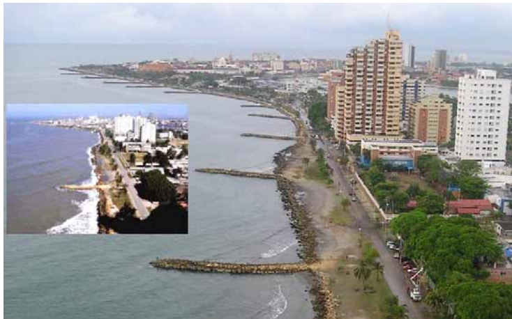
Figure 6. Overview of the hard structures constructed along the Bocagrande sector between 1999 and 2004.
